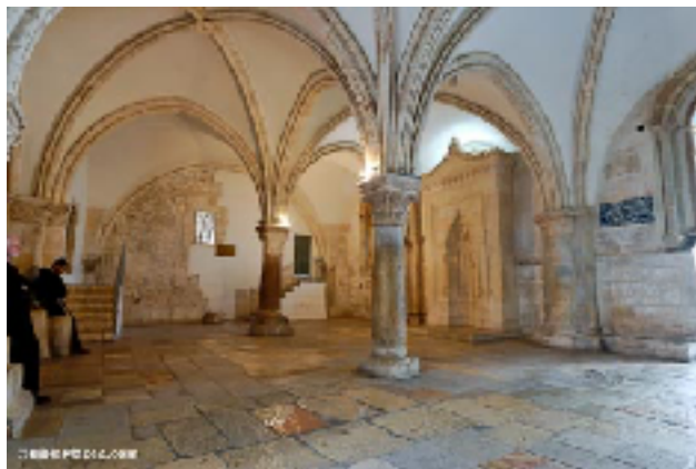
Air space of the Upper Room
